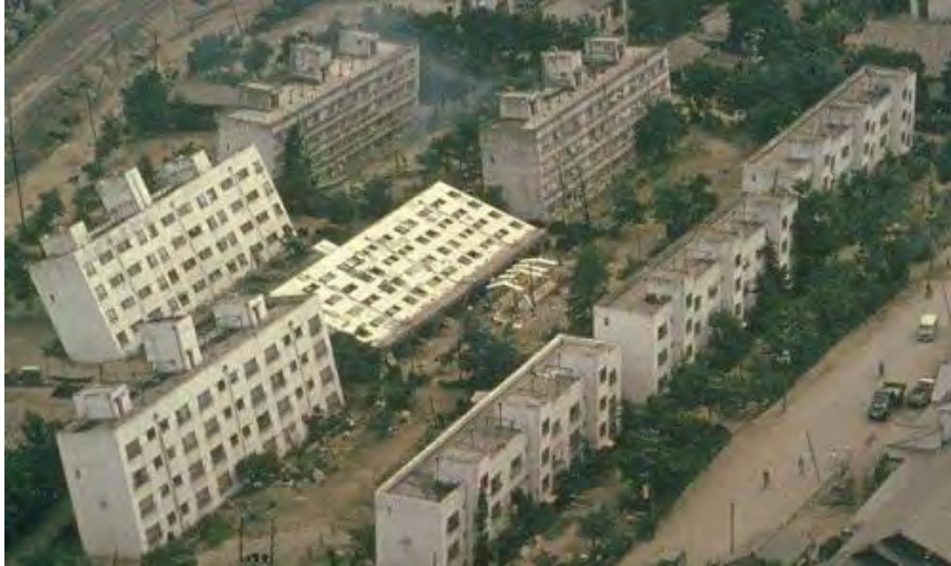
Some effects of liquefaction after the 1964 Niigata earthquake (Source: Wikipedia)
