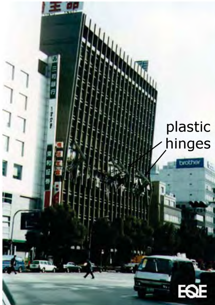
Mid-story collapse, 1995 Kobe earthquake (EQE Summary Rep., 1995)
