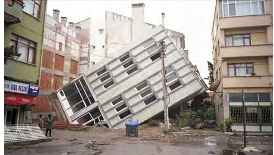
Foundation Weakening Due to Soil Liquefaction after 1999 Adapazari earthquake, Turkey (Source: USGS)
